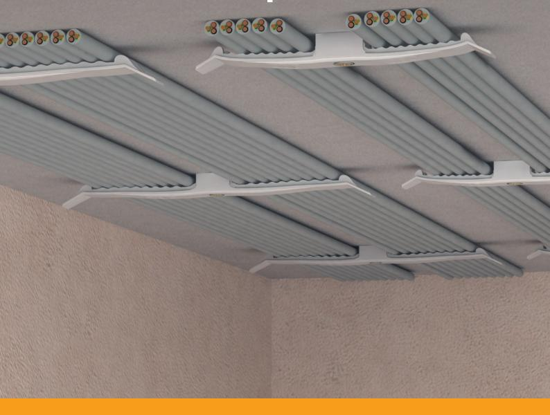
The installation variant with the the pressure clips is particularly ideal when there is little installation height available under the ceiling, for example for use on intermediate ceilings and partition walls. With the small installation dimensions, fire alarm cables and small power cables for safety lighting systems, for example,
